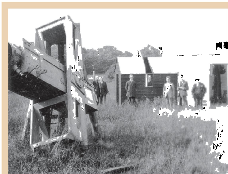
Figure 3. Instrument no. 3: 18-inch mirror by George H. With, presented by N. E. Green in 1897. Here it is set up in a wooden mount in the rectory glebe of the Rev T. E. R. Phillips at Headley, Surrey. The photograph was taken around 1930, during one of Phillips’ Annual Visitations. (RAS MS Phillips 5B; copyright Parish of Headley.)
