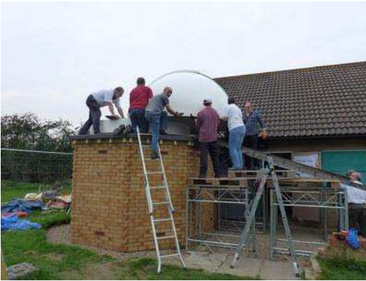
Members of CMHAS erecting the dome.
