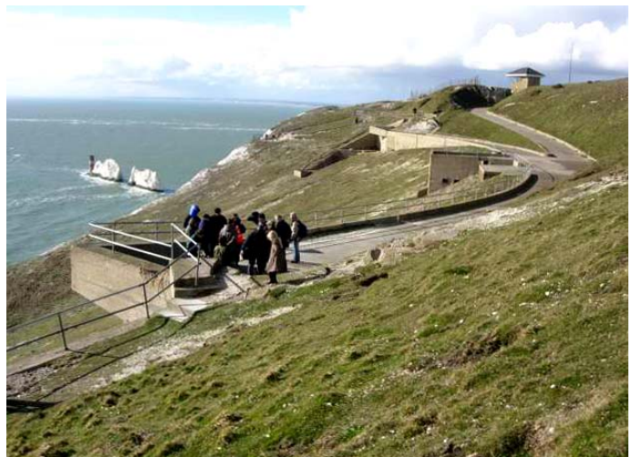
The former rocket testing site at the Needles Battery. Photo: S. J. Griffiths
