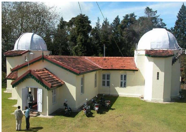
Kodaikánal Observatory's first building, dating from 1899. Photograph courtesy Rajeev Singh.
