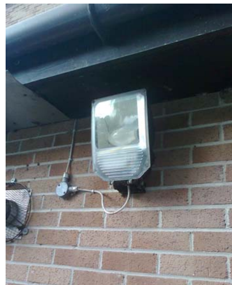
Example of a ‘rottweiler’ light set at the wrong angle. If used at all, such a unit should be mounted with the glass almost parallel to the ground. (Bob Mizon)
