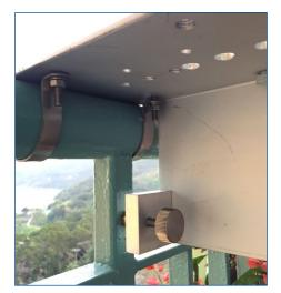
The mounting bracket. Note how it is clamped and stabilised without the drilling of any holes in the balcony.
