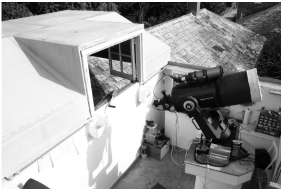
Figure 1. View of observatory with roof rolled back.
