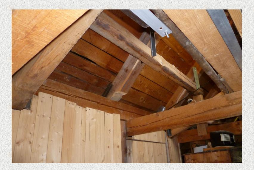
Tripod stands by one leg on the wall others legs stand on beam which is not connected with floor.
