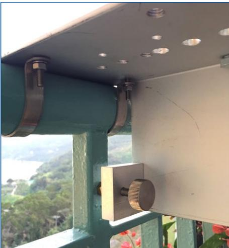
The mounting bracket. Note how it is clamped and stabilised without the drilling of any holes in the balcony.
