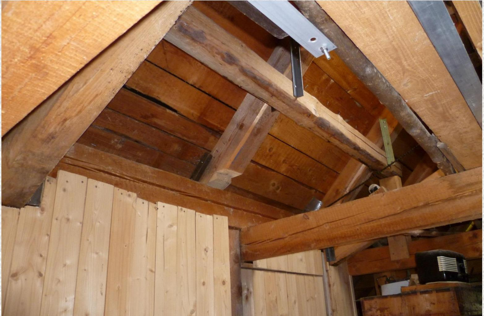
Tripod stands by one leg on the wall others legs stand on beam which is not connected with floor.
