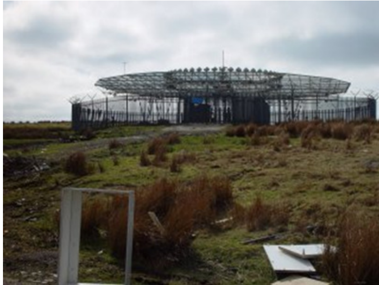
Figure 3 The Brecon VOR Beacon
