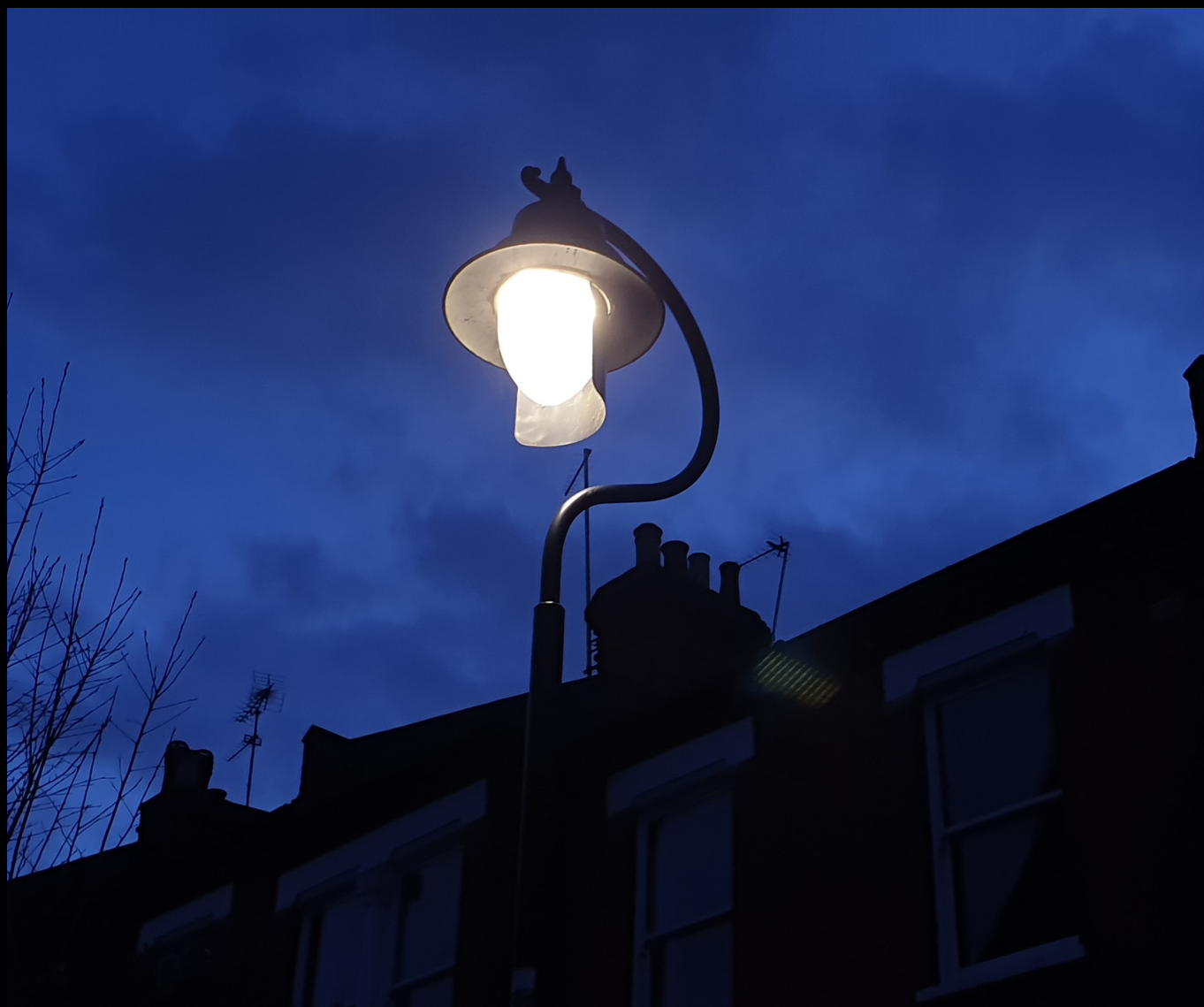
Shielded streetlight in residential context
