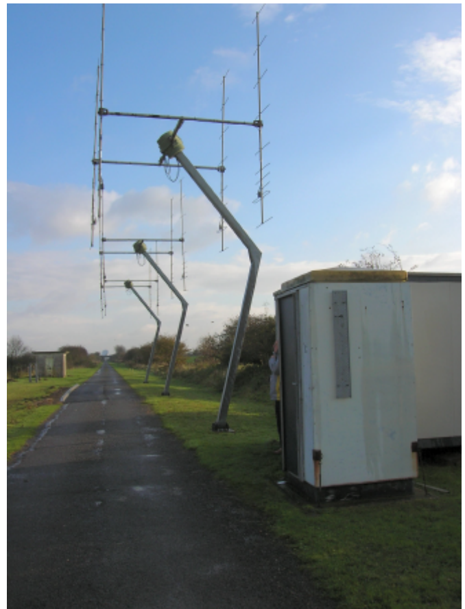
Aerial arrays 4, 5 and 6, and the receiver cabin, just in front of the BAA Hut
