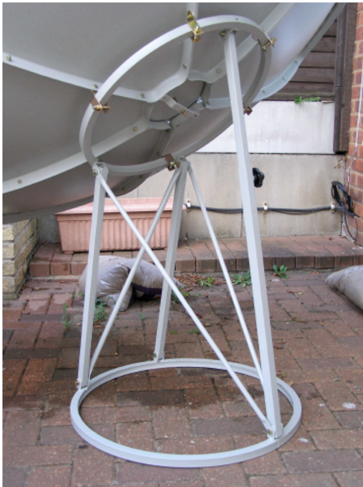
The dish mounting assembly
