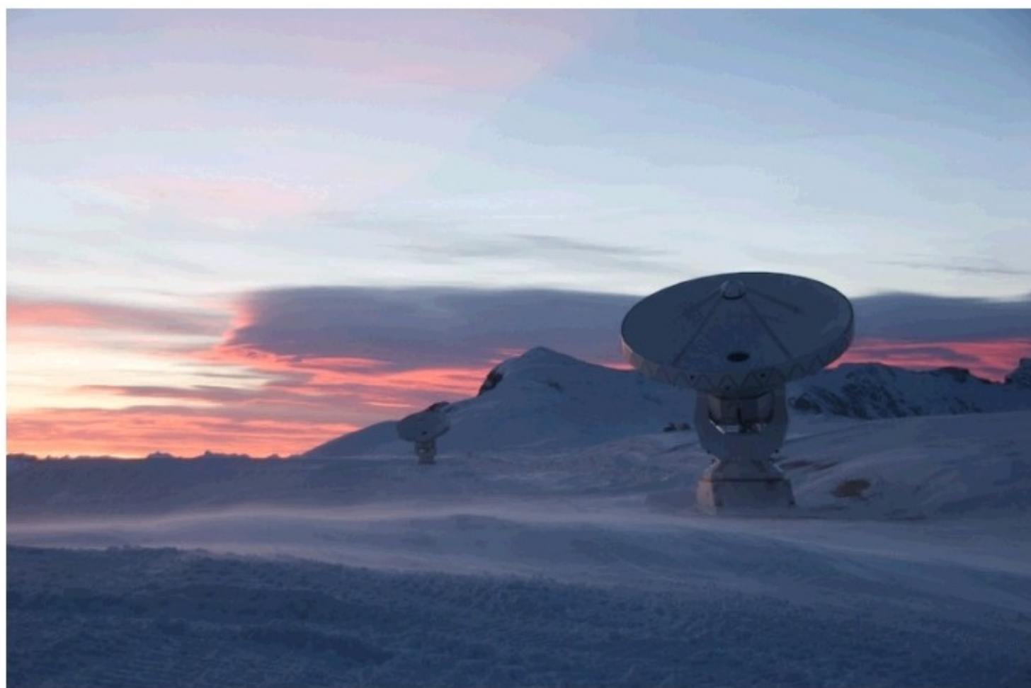
Photo: Sunrise on the Plateau de Bure, showing two of the six 15 m dia. mm-wave antennas 2,550 m up on the Hautes-Alpes. Courtesy of IRAM
