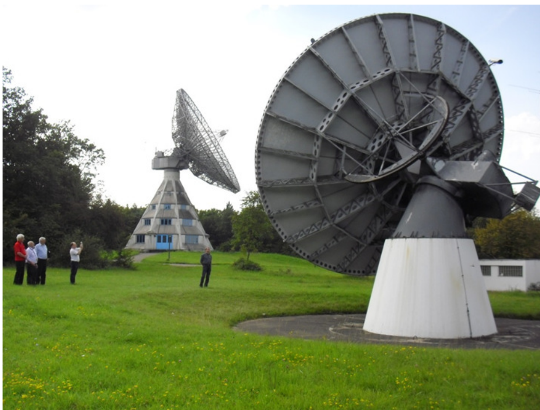
Astroteiler Stockert, showing the original 25 metre dish and observatory, with the later 10-metre diameter solar instrument in the foreground.
