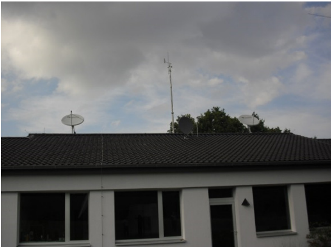
The 1.2 m dishes used in the interferometer
