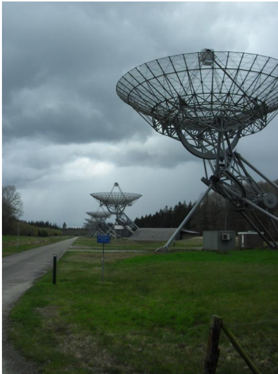
(Figure 4 A few of the fixed-position 25 m dishes that form part of the WSRT. Four other dishes are mounted on railway tracks)
