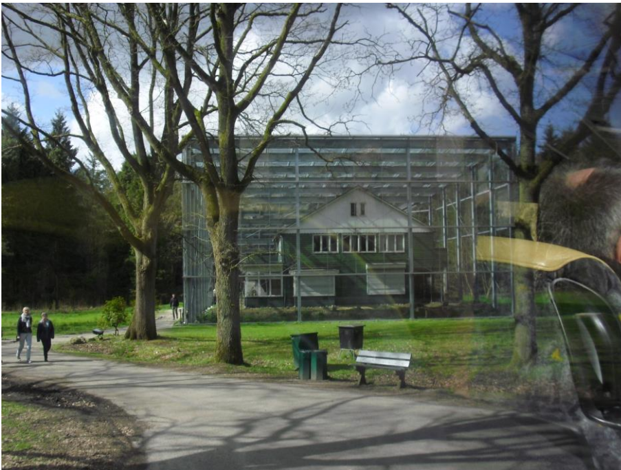
(Figure 9 The Camp Commandant's house, part of the memorial museum. A 200-seat auditorium has been included at the rear, all enclosed within this huge glass structure.)
